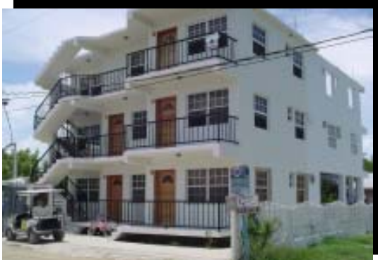
BEST DEAL ON THE ISLAND. BRAND NEW ONE BEDROOM CONDO LOCATED ON THE THIRD FLOOR WITH INCREDIBLE VIEWS FACING THE OCEAN. OPEN FLOOR PLAN WITH OVER $6000 IN NEW FURNITURE AND SPLIT UNIT 12,000
